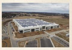
Gold Certification. Of which, the most notable feature is the 865 kW Photo Voltaic solar array that covers over 90% of the roof (as seen in the photo to the right). The array generates approximately 50% of the buildings annual energy.
