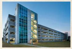
The building is a six story blast-rated office building, meaning the structure can withstand an explosive attack. The building's skin is comprised of blast-hardened architectural precast concrete with
